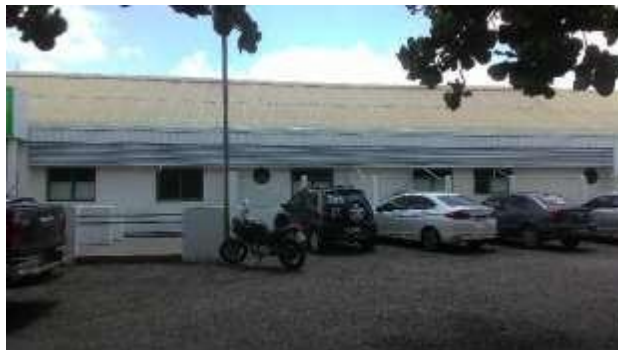
Grades fachada principal
