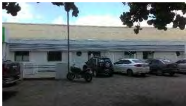
Grades fachada principal
